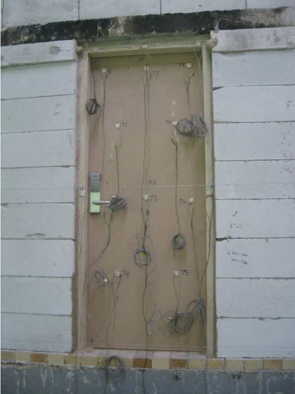
Fig. 3 - Unexposed Side Prior to the Fire Test
