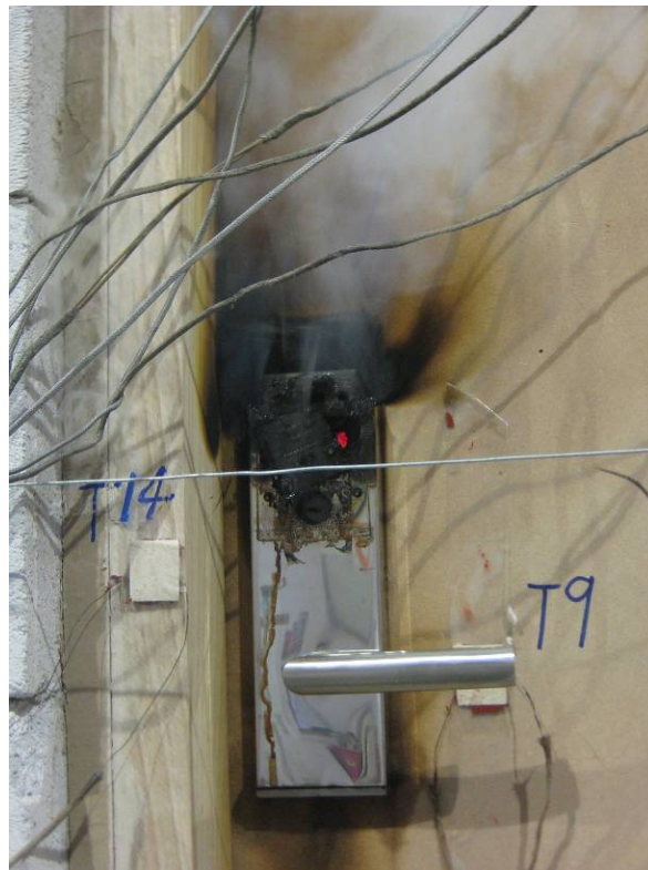
Fig. 6 – Unexposed Side after 25 Minutes
