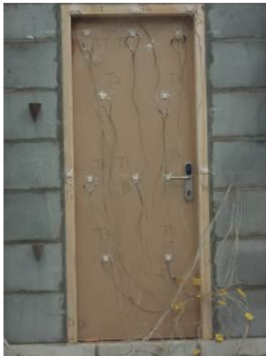
Fig. 4 – Unexposed Side after 10 Minutes
