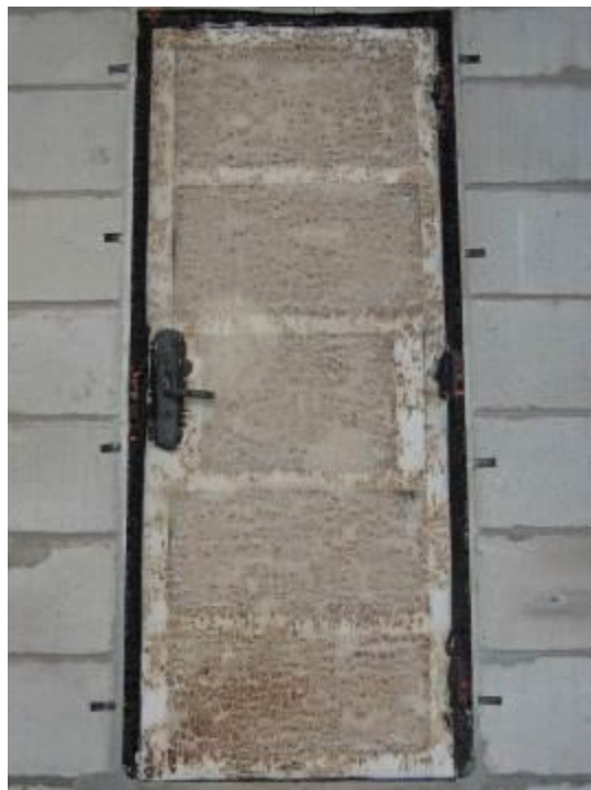
Fig. 10 –Exposed Side after 60 Minutes
